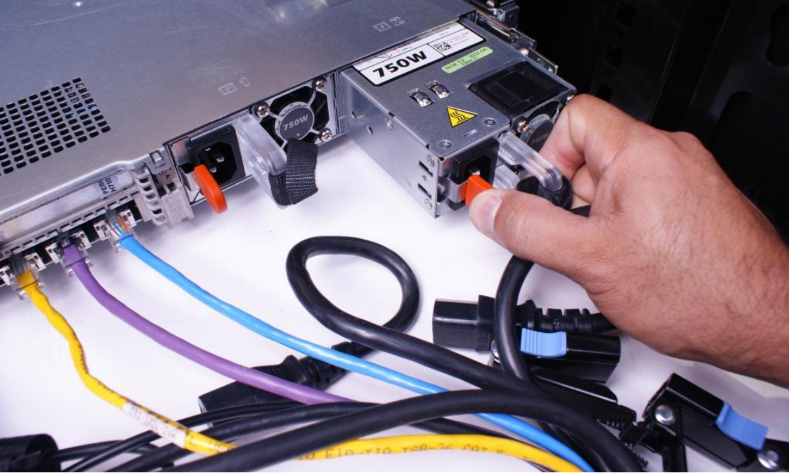
Figure 8. Replacing the outer power supply
