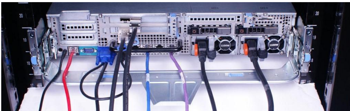
Figure 1. System with cables installed
