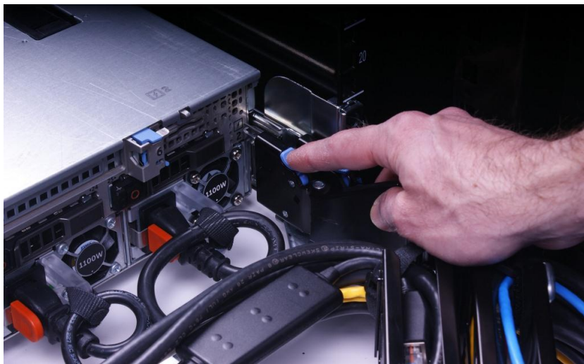
Figure 7. Disconnecting the CMA attachment housings
