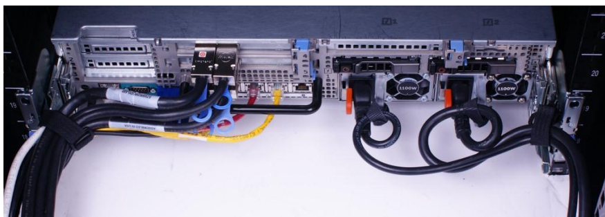
Figure 9. Cable routing without a CMA
