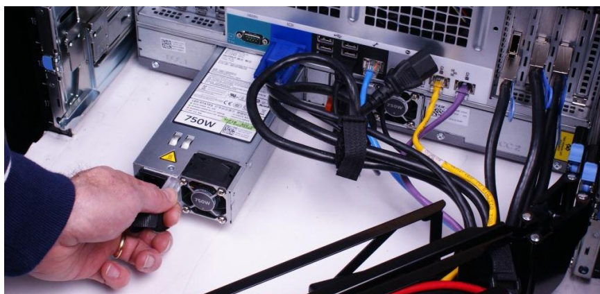
Figure 6. Replacing the power supply
