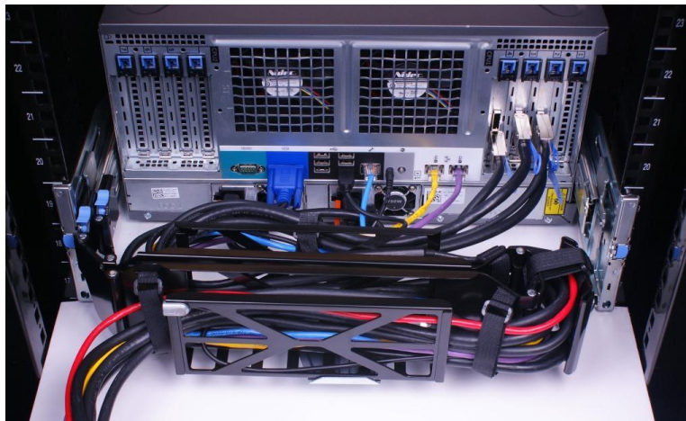
Figure 5. Right-side mounted CMA installation
