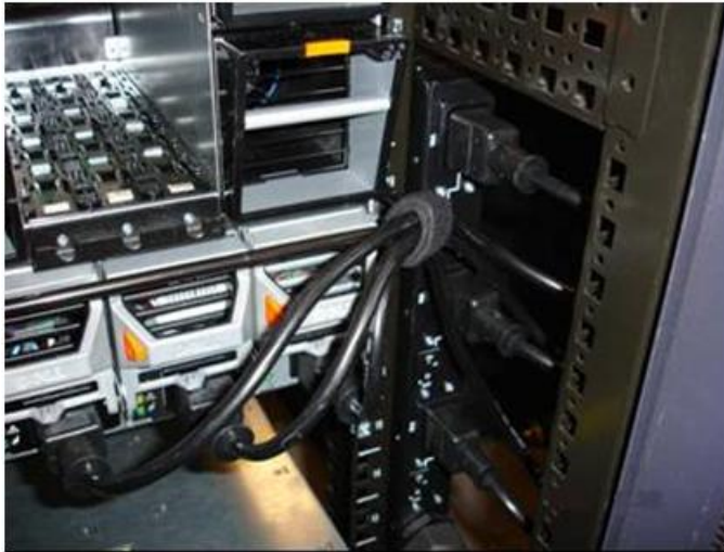
Figure 2 – The 24 Amp Three-Phase PDU connected to Power Supply Units. The 48 Amp Single-Phase PDU (not shown) is connected in the same manner. Note that the jumper power cords are secured to the system strain relief bar.
