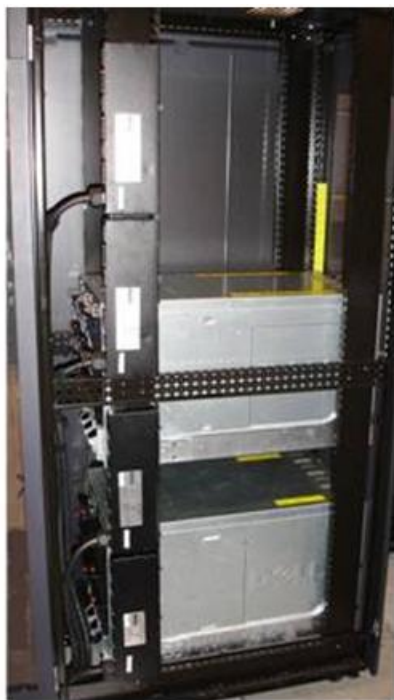
Figure 5 – Mounting of four PDUs in the 0-U Space of the Dell 4210 Rack.
