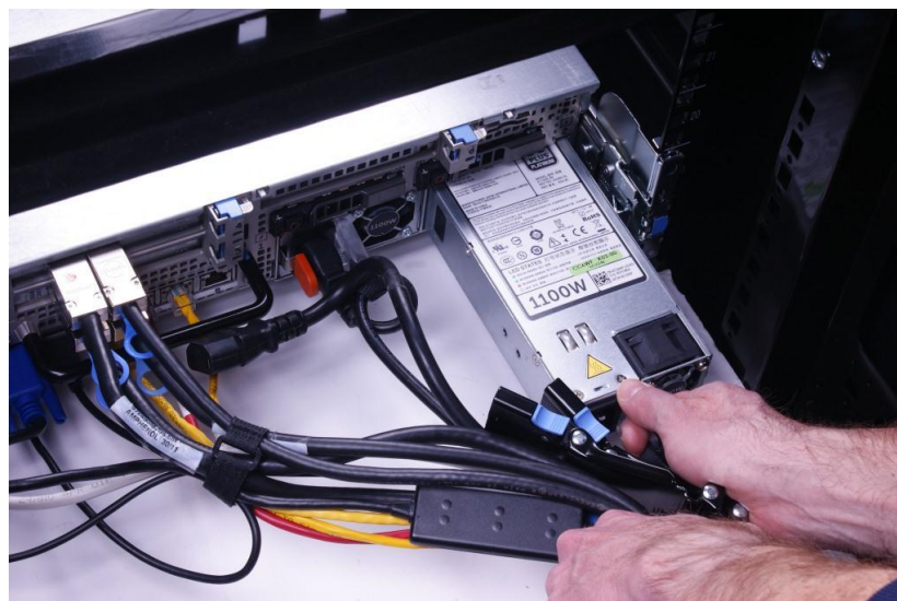
Figure 8. Replacing the outer power supply
