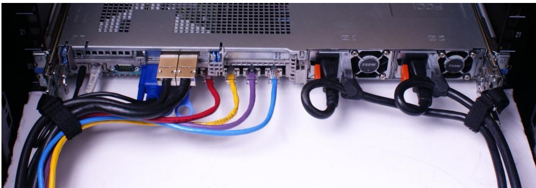
Figure 9. Cable routing without a CMA
