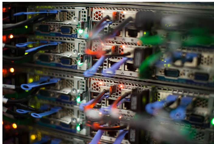
Figure 2. Optimized racking and cabling for high density, servicing, reliability and redundancy
