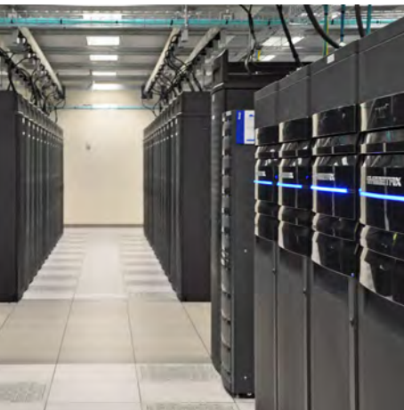
EMC Durham Data Center
