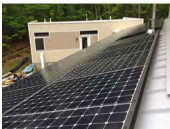
EMC employee Mark Stephan installed 27 solar panels on the roof of his newly constructed home through the EMC Home Solar program.
