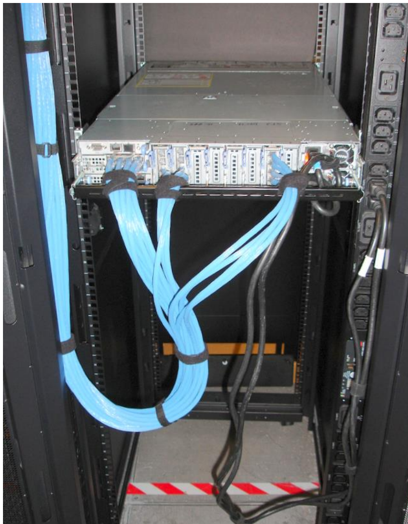
Figure 6. System with cables secured to SRB in rack
